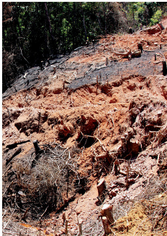
Ecosystem-services loss, and geo-hidrologic processes arising, by erosion and sediment deposition in watercourse. Implementation of the North Ring-Road, Guarulhos region (São Paulo/ Brazil), with deforestation, and processes of cut and landfill. Photograph: Antonio Manoel dos Santos Oliveira, 2014
